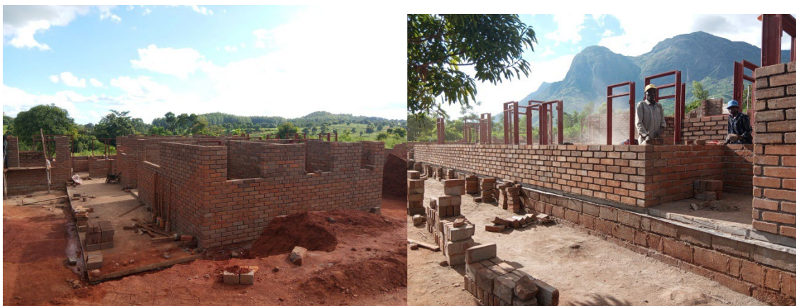
Figure 4: Inde Mulanje processing facility under construction in Mulanje
